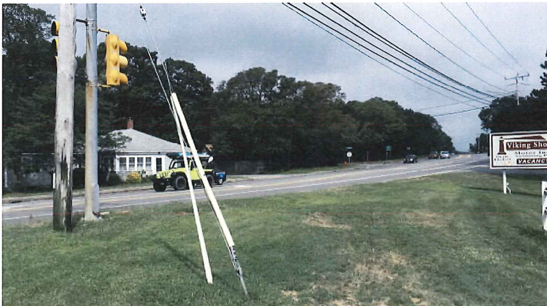
Figure 14 – Potential sight obstructions in northeast quadrant of Nauset Road intersection - utility pole and guy wires
