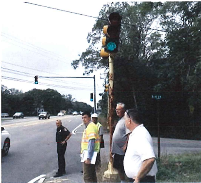
Figure 7 - Route 6 southbound signal housing damaged and tilting
