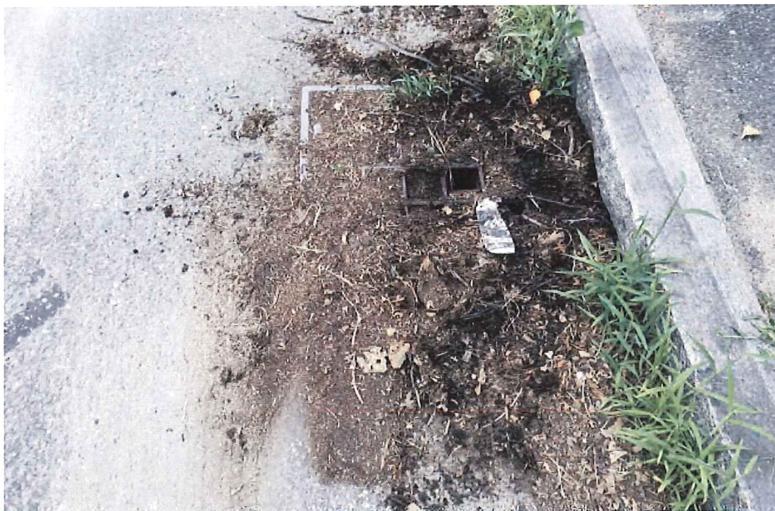
Figure 15 - Catch basin blocked by debris
