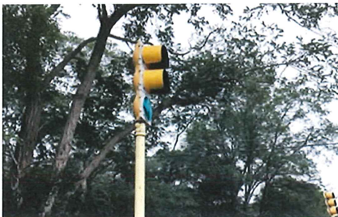
Figure 8 - Entrance to Wampum Lane green signal head missing visor
