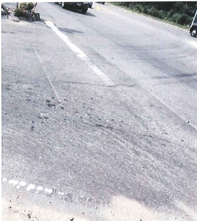
Figure 11 - Stop bar worn at Nauset Road approach
